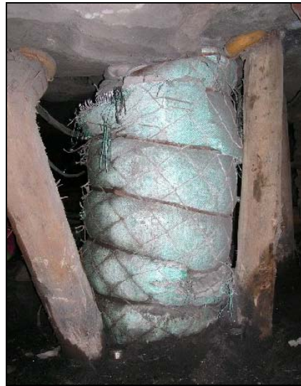
Figure 6.9 550 mm RSS pack with 150 mm closure at the Spud shaft site
