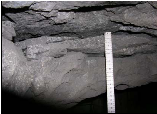
Figure 6.2 Low angle fractures throughout the panel
