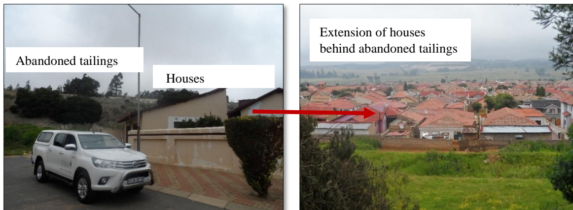
Figure 37: Extensive unprotected tailings which cover a large area nearby residential areas and therefore could affect health status of individuals residing nearby through the dust blown from these sites.
