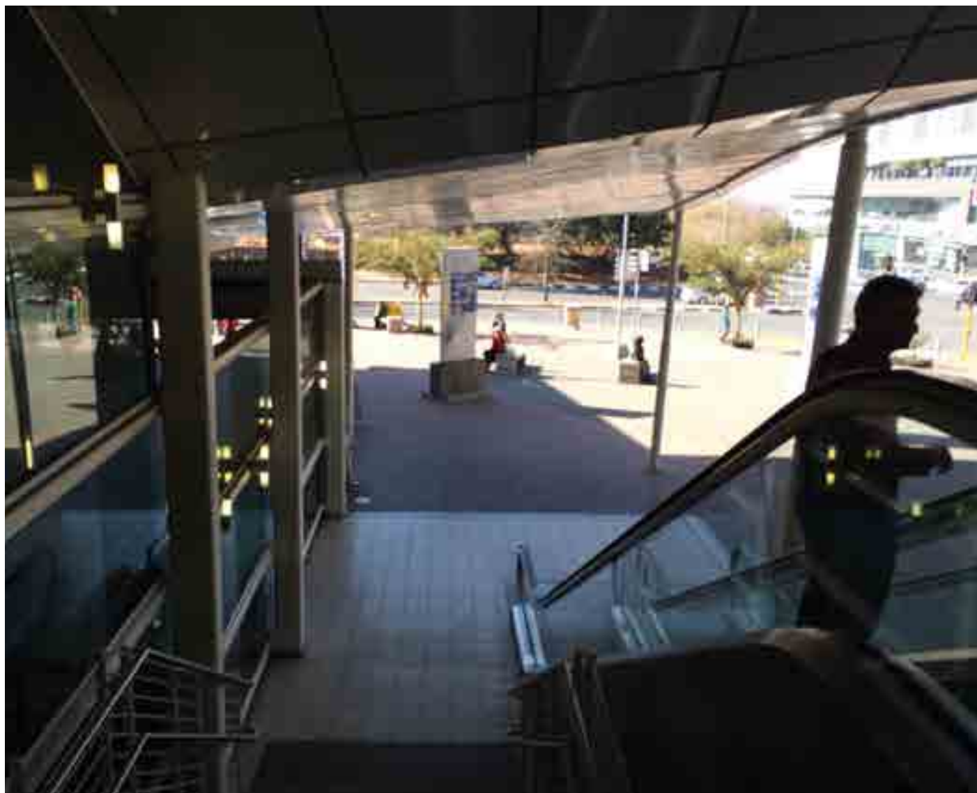
Figure 4.10: Sandton Station entrance (L). Escalator from the Sandton station to the phase 2 podium level above (R). (Source: Guy Trangoš)
