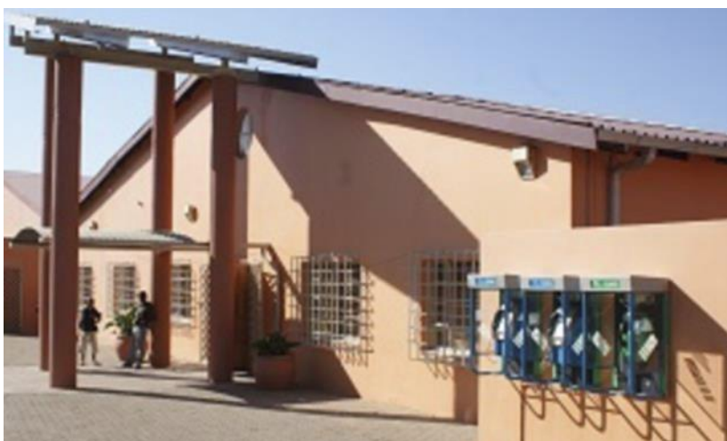
Figure 6 is a photograph of the Mofolo recreational centre in Soweto.
