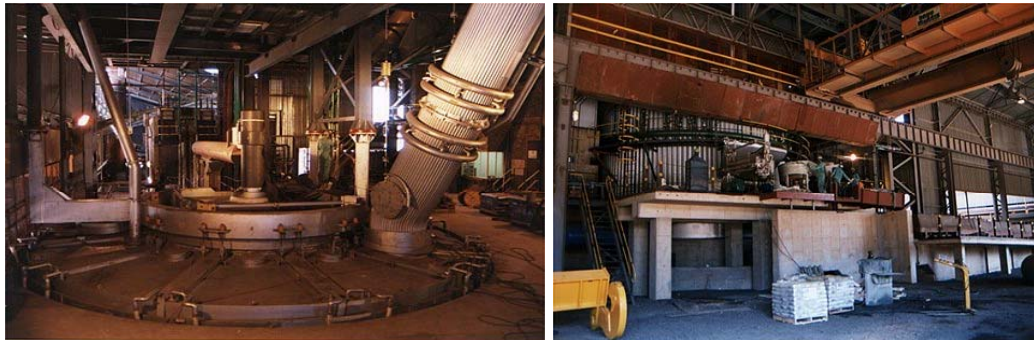
Figure 2.10 Middelburg Ferrochrome built a 44 MW (62 MVA) DC arc Furnace in Middelburg in 1997
