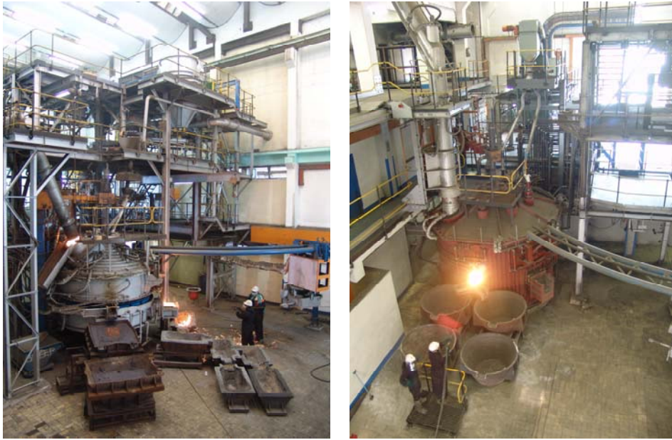
Figure 2.23 1.5 MW and 3 MW DC arc furnaces at Mintek
