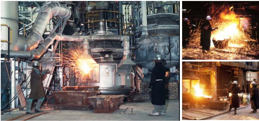
Figure 2.12 Ilmenite smelting testwork at Mintek
