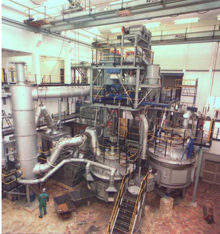
Figure 2.24 5.6 MVA DC arc zinc fuming furnace pilot plant at Mintek
