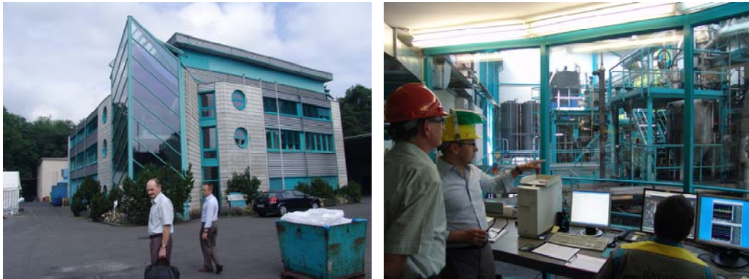
Figure 2.18 Batrec battery recycling plant in Switzerland
