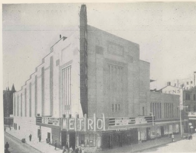
entrance at the corner of bree and hoek streets.
