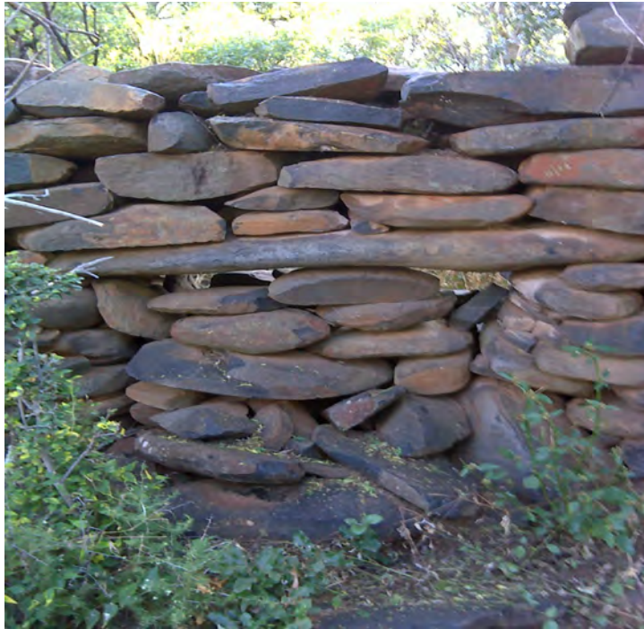
Figure 5.7: A sealed lintel in the north eastern anomalous kraal
