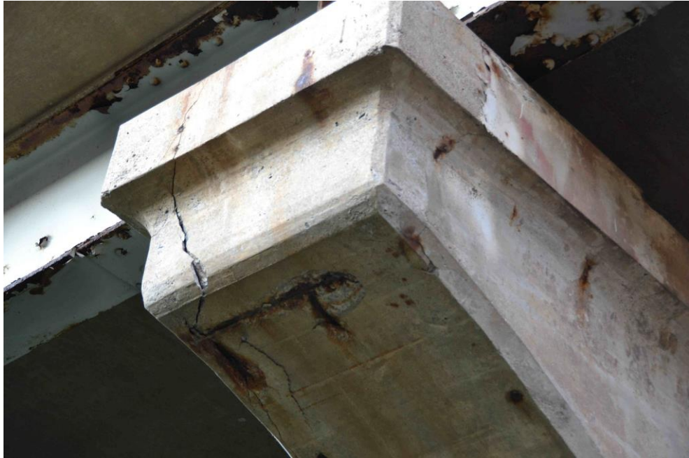
Figure 2: “Rust in reinforced steel.” WikiCommons image. Creative Commons License. (Accessed November 28, 2022. https://upload.wikimedia.org/wikipedia/commons/thumb/4/43/Qew_bruecke_nf_beton_kaputt_33_von_46.jpg/2560px-Qew_bruecke_nf_beton_kaputt_33_von_46.jpg )
