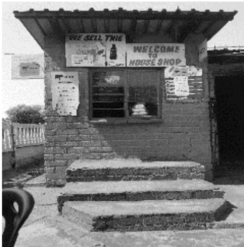
Photograph 4: Second Structure of Tuckshop
