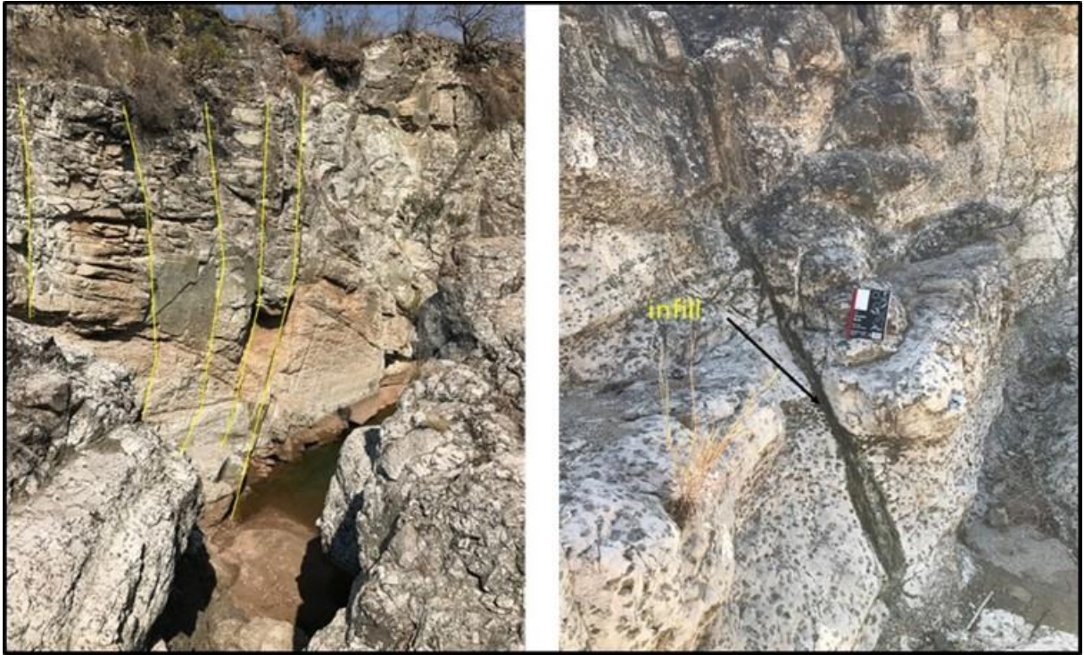
Figure 23: Major joints striking in an N-S direction on the Tweefontein farm, the joint on the right has secondary mineral infill (biotite and chlorite).
