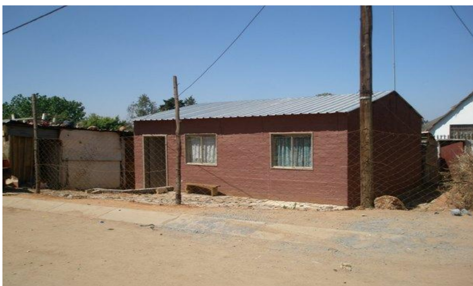
Figure 5: Zandspruit Transit Camp Housing. Source: (Ole Saibul, 2008)
