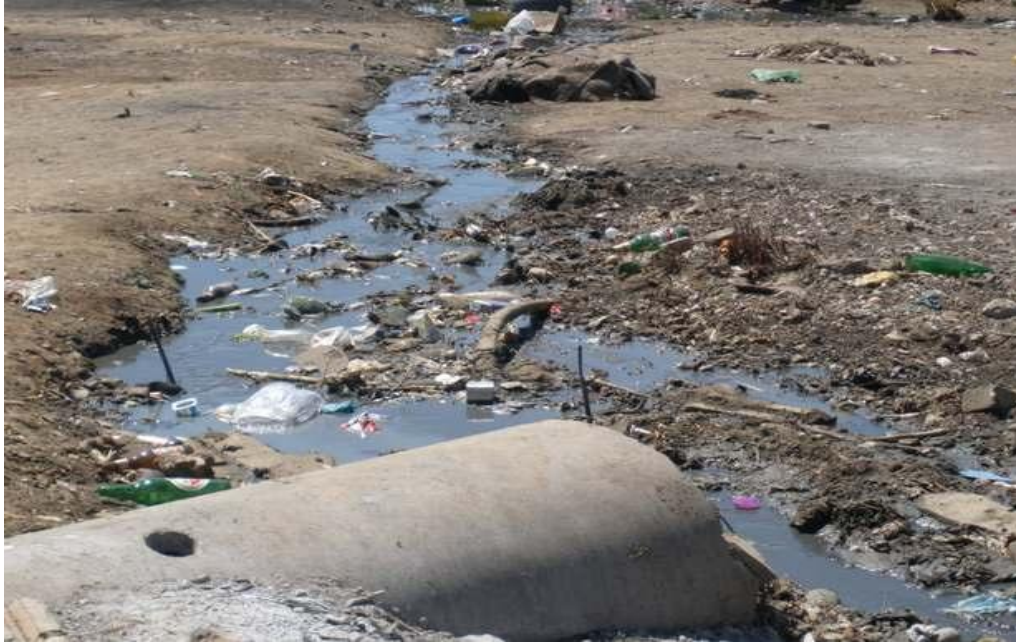
Figure 13: Lack of services in Zandspruit Private Property (no drainage).
