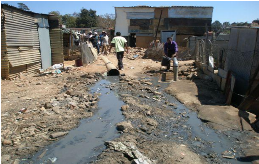
Figure 12: Lack of services in Zandspruit Private Property (no drainage). Source: (Ole Saibul, 2008)
