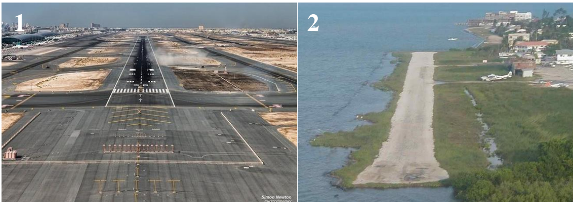
Figure 2-1: Comparison between prepared and unprepared runways. 1 - Prepared runway at Dubai International Airport with visible markings and landing lights [3]. 2 - Unprepared runway in Belize showing no markings and lights [4].
