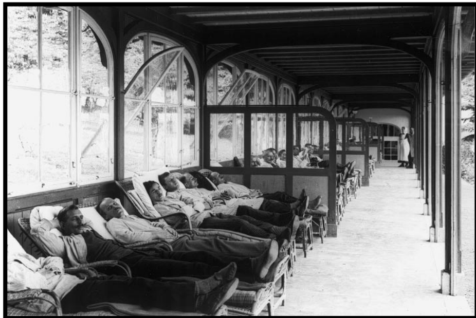
Figure 1.2 TB-infected patients resting on cane recliners, with moderated sunlight, in a sanatorium (1892). This image represents the BASF sanatorium for consumptives (Dannenfels, German. BASF Aktiengesellschaft, BASF AG).(Source: Campbell M. What tuberculosis did for modernism: The influence of a curative environment on modernist design and architecture. Med His. 2005;49(4):463).
