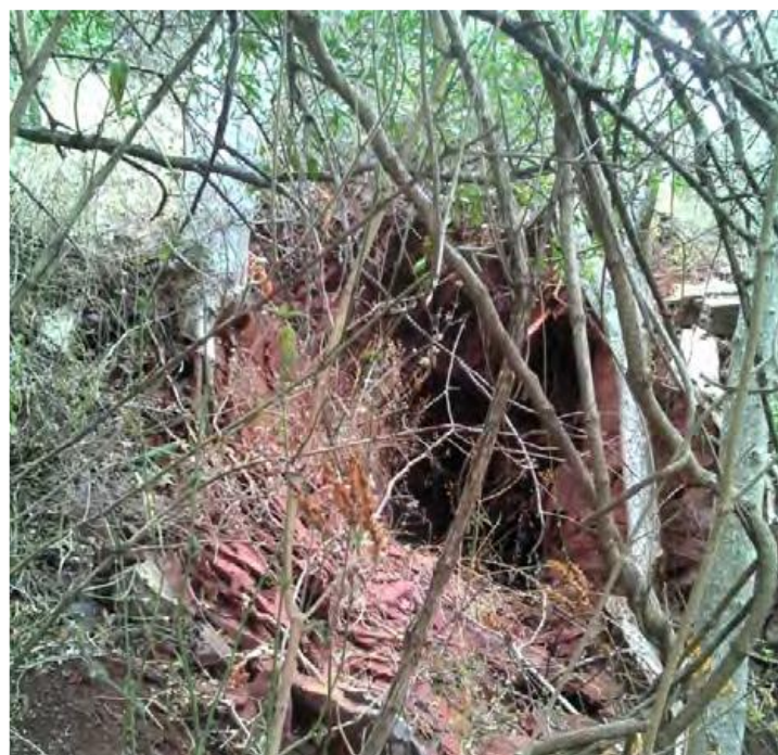
Figure A-3.2: Adits are small, usually hand-dug inclined or horizontal entrances to asbestos seams that are found on most project sites (Source: Author)
