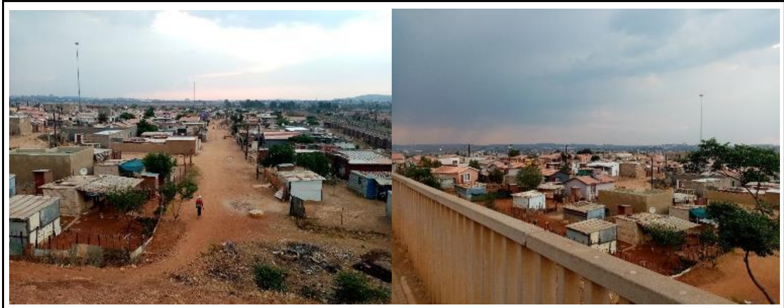
Figure 4.6: Pictures of structures on area of study Source: own images, taken October 2019
