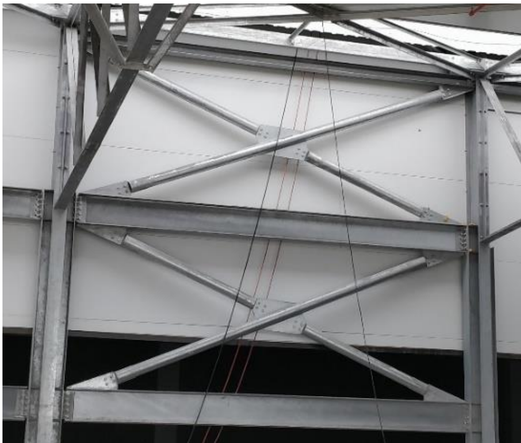
Figure 4-6 Site A Cross-braced CHS Configuration (Site A-C2)
