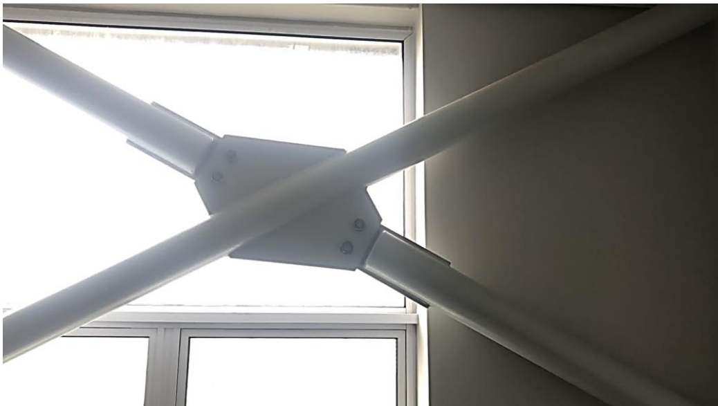
Figure 4-7 Site B Cross-braced CHS Configuration (Site B-C1)
