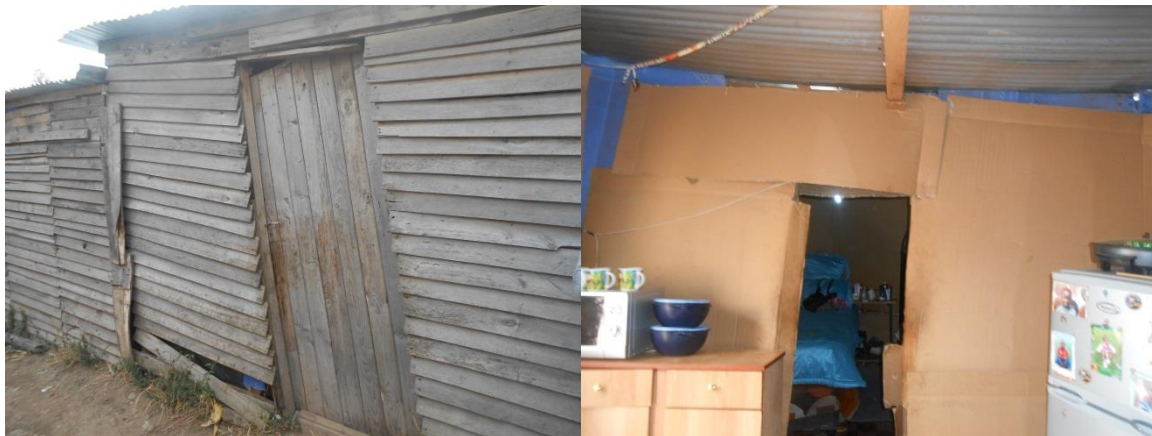
Image 1: The external (made of wood) and internal (lined with cardboard) parts of the shack where I stayed during my research at Ford Street, Duncan Village: Photo by Patricia -1/08/2014.
