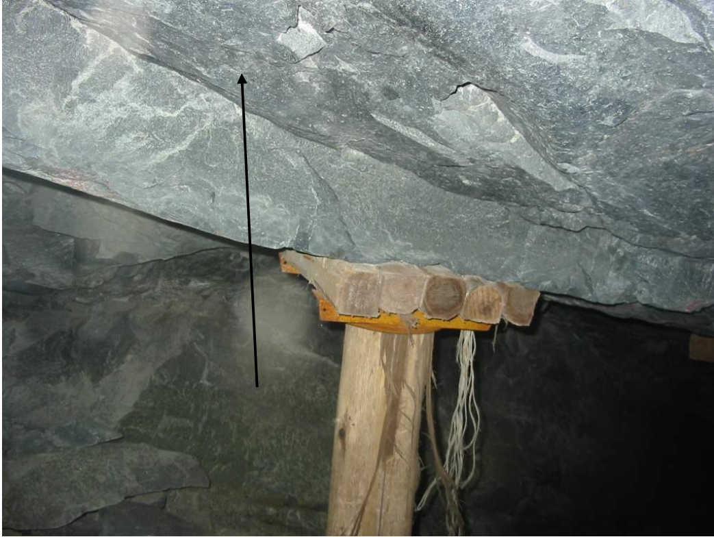
Figure 3.4b Joint planes in stope hangingwall
