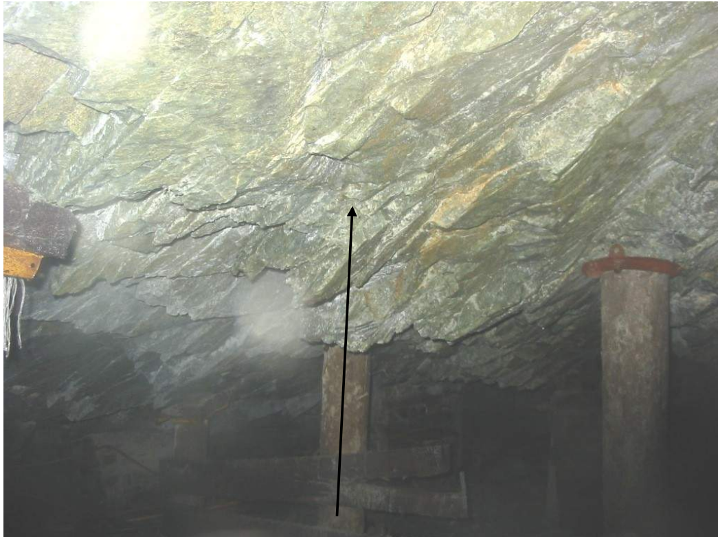
Figure 3.5b Stress- induced fractures in stopes
