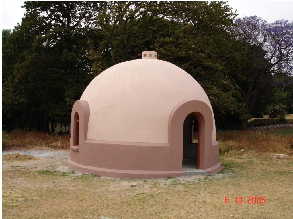
Figure 1.2: A completed thin shell low-cost housing structure (Gohnert n.d.)
