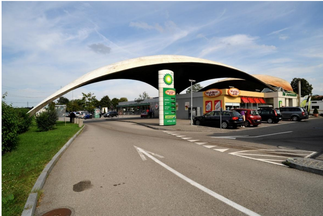
Figure 2.10: Heinz Isler's motorway service station in Deitingen ( commons.wikimedia.org )
