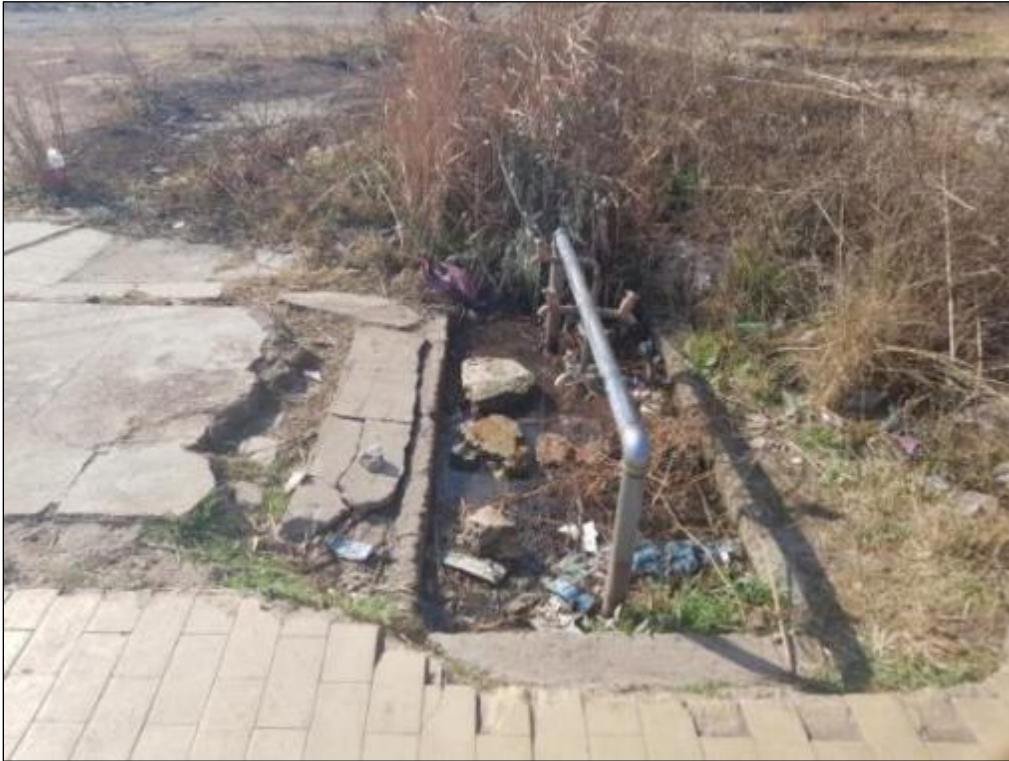
Figure 3.6 Residents of Bottom Compound are supplied with water from communal stand pipes. (Author's photograph, 18 August 2021)
