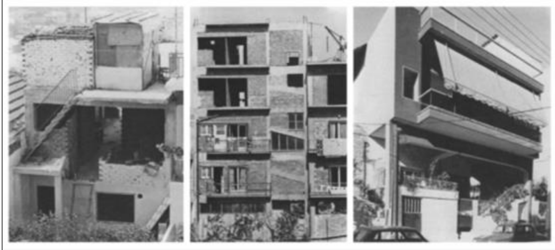
Figure 4.7 Examples of incremental concrete frame construction adding additional floors ( 'panosikoma' ) to self-built houses on the periphery of Athens. (Source: Dimitris Philippides, 1984) (Found in Magouliotis, N., 2018: 5)
