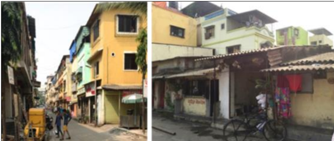
Figure 4.6 Incremental housing in Mumbai showing densification of one-room houses on small stands (right) into double-storey houses (left). (Photography by Sumila Gulyani) (Source: World Bank)
