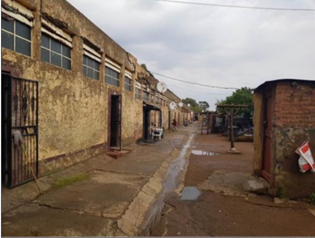
Figure 4.1 Bottom Compound on a rainy morning. (Author's photograph, 1 October 2021)
