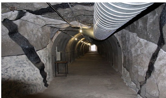
FIGURE 8 Wits mock mine tunnel.
