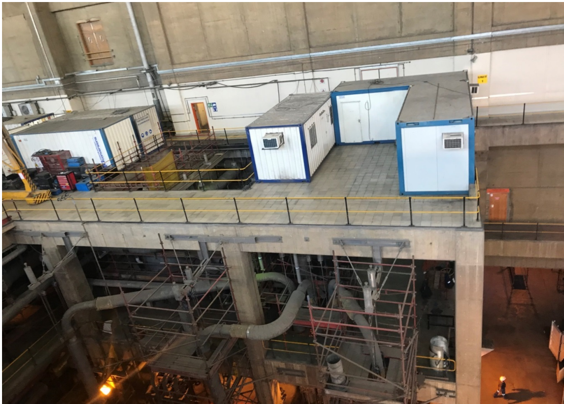
Figure 47: Containers placed next to the unit – this area could have been utilised for storage of heavy components.
