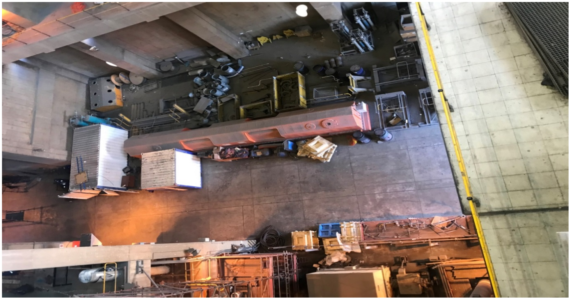
Figure 49: Basement of the unit showing storage space that can be utilised more effectively.
