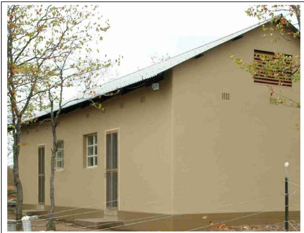
Figure 3.3 Example of the buildings painted in the Kruger Park iconic khaki
