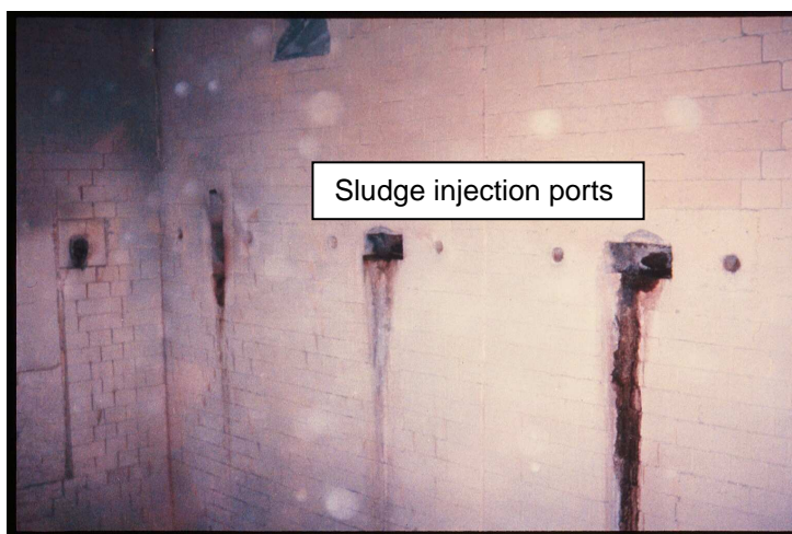
Figure 4.18 Sludge injection wall, of the sludge and coal co-fired FBC
