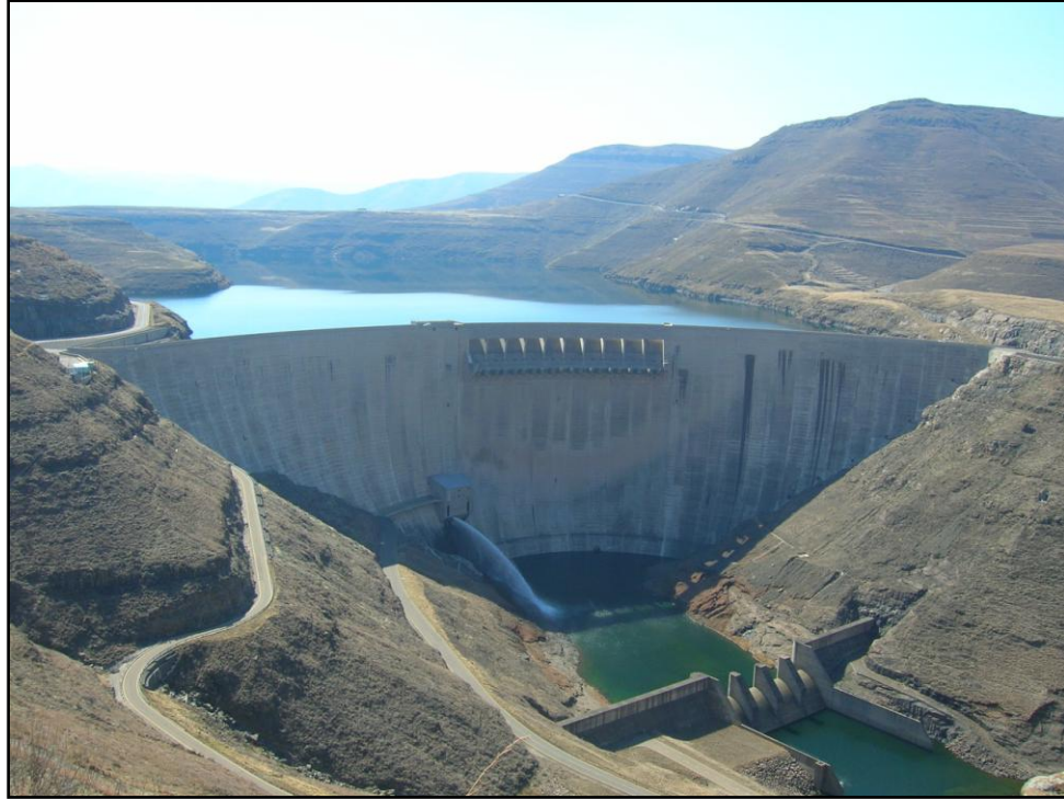
Photo 2 : The Katse Dam wall. Katse Dam is the highest double curvature dam in Africa.
