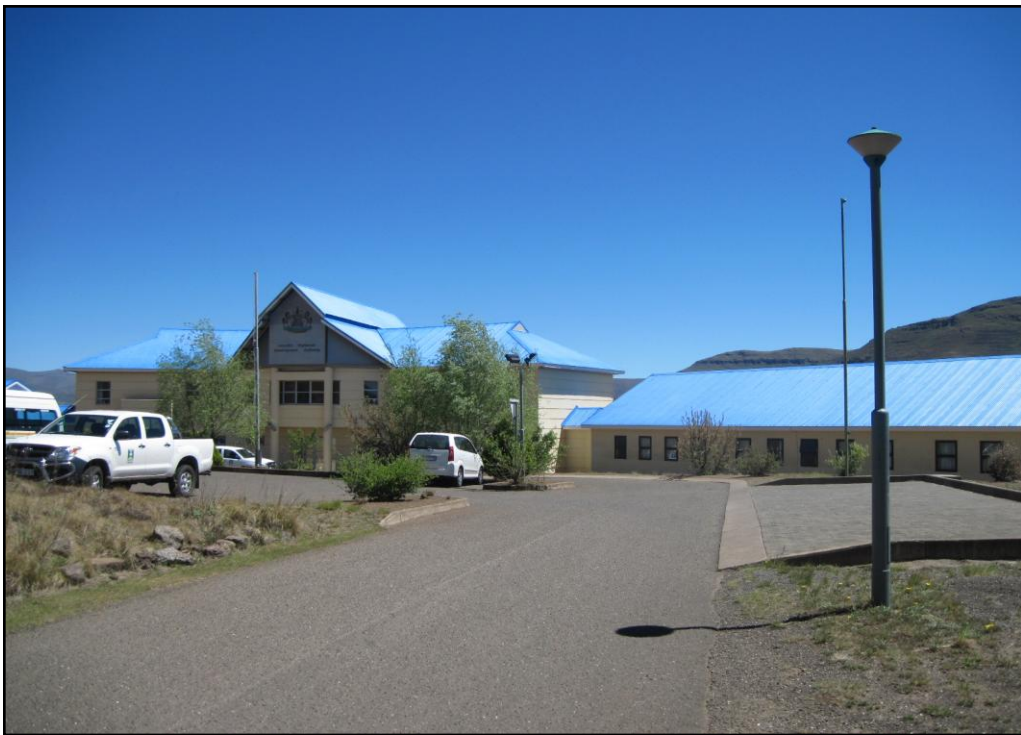
Photo 6: LHDA headquarters in Katse.
