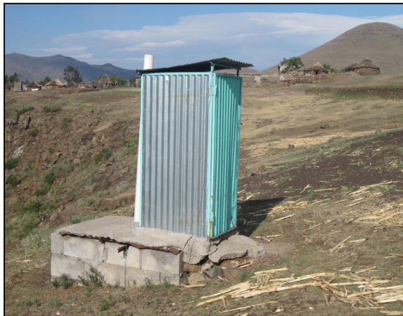
Photo 8: A ventilated pit latrine constructed by LHDA in Khohlo-Ntso in the early to mid-1990s, remnants of the water sanitation project under the LHRF.
