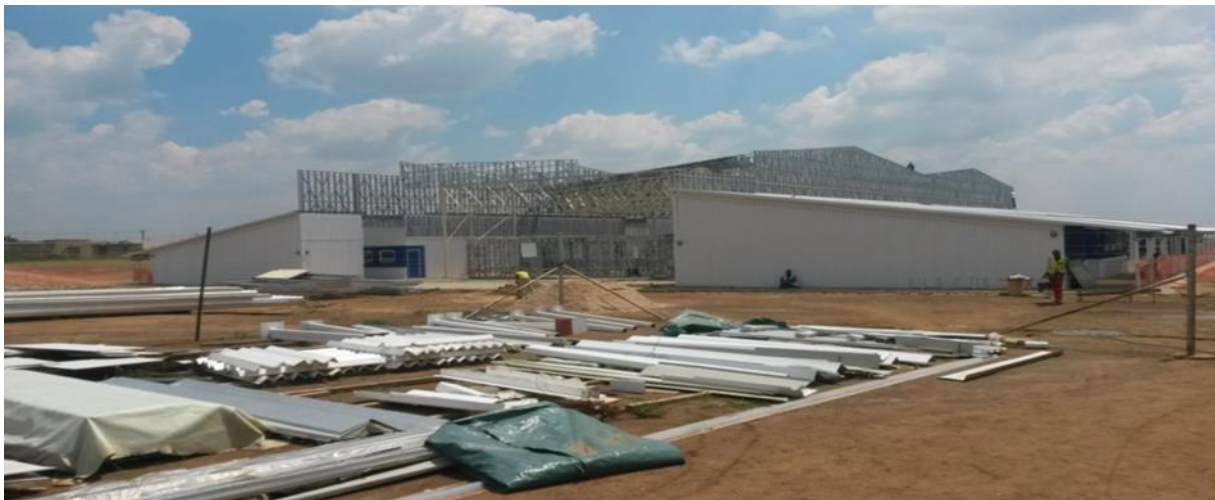
Figure 5: Picture of a school in construction in Tsakane (East rand)
