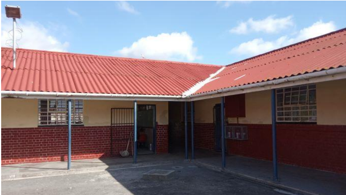
Figure 7.3 Exterior walls of Grade 6, Grade 7 and Grade 5 classrooms
