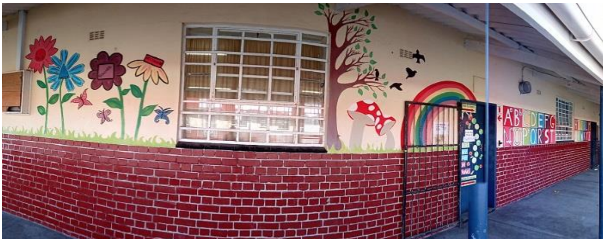
Figure 7.2 Exterior walls of Grade R and 3 classrooms
