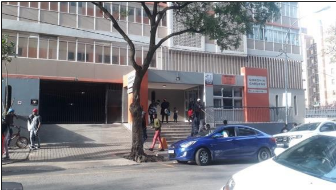
Figure 3.12: Street view of Corona Gardens (Source: Resident D's photograph, 17 December 2021)
