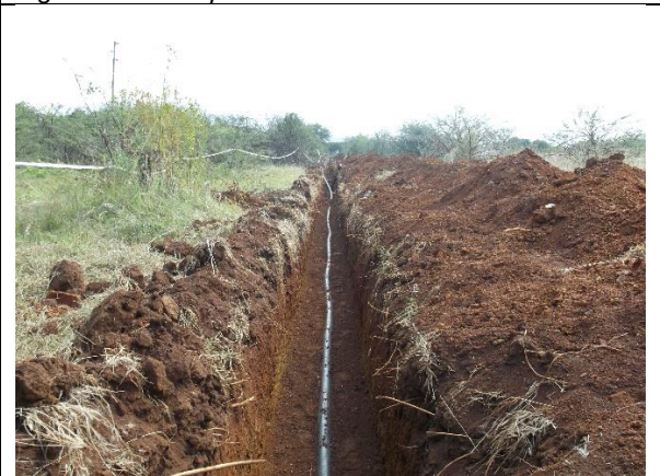
Figure 4.6 : Water main line during construction
