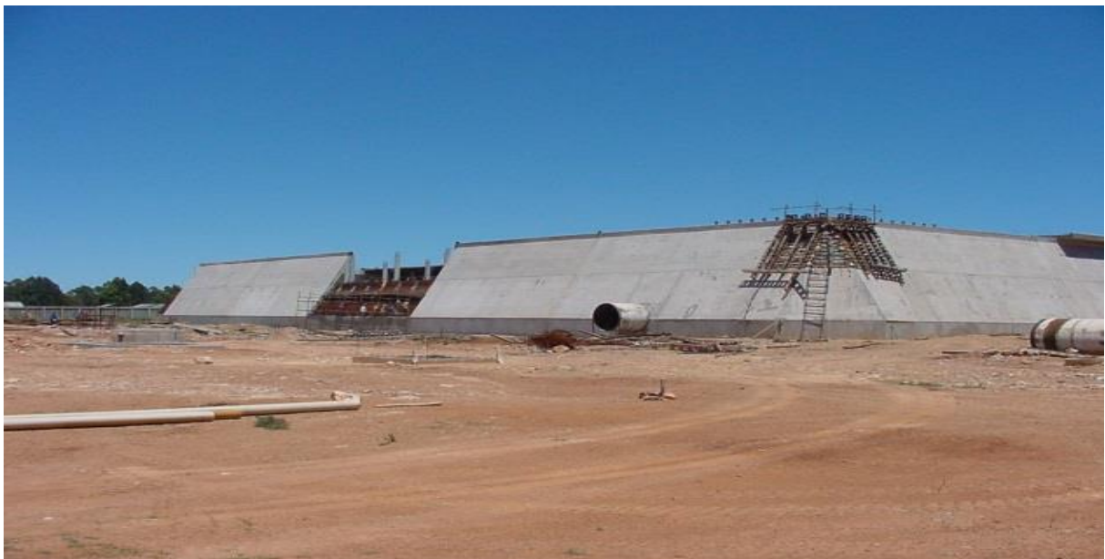
Figure 2.6: Daleside reservoir without the embankment, wall construction
