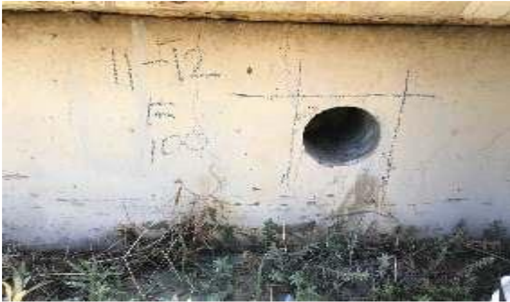
Figure 3.7: Typical 100mm diameter core out of test reservoir
