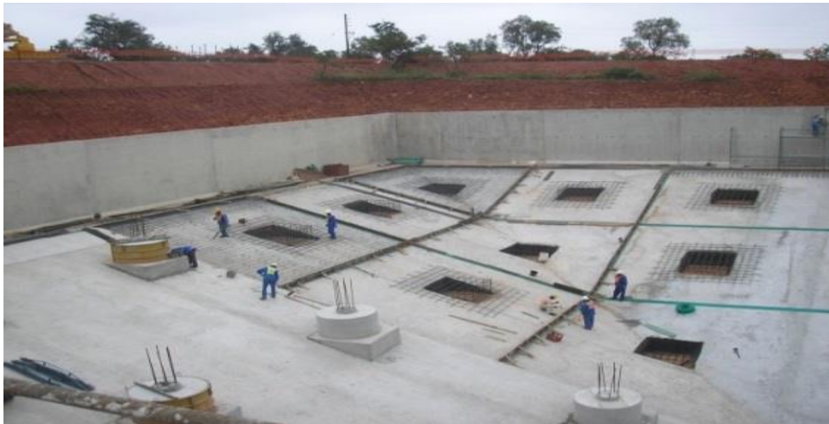
Figure 2.7: Construction of Rustenburg reservoir
