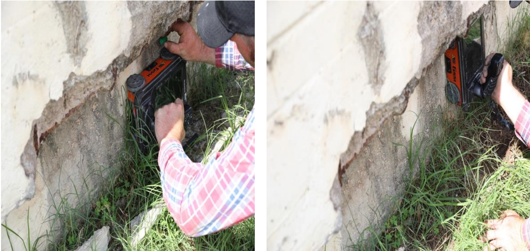
Figure 3.8: In-situ cover depth survey using a cover meter
