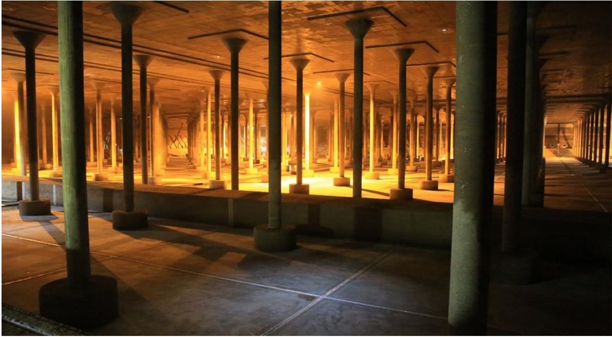
Figure 3.1: Typical interior of a Rand Water reservoir
