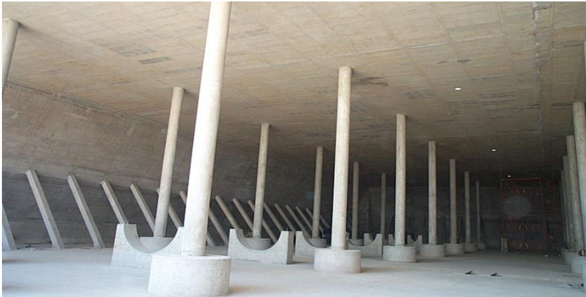
Figure 2.8: Typical internal configurations for Rand Water reservoir
