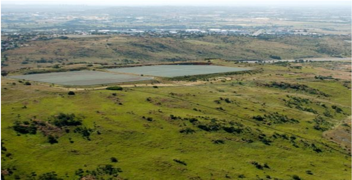
Figure 2.5: Klipriviersberg reservoirs buried, 13.5m into the ground and 20m apart
