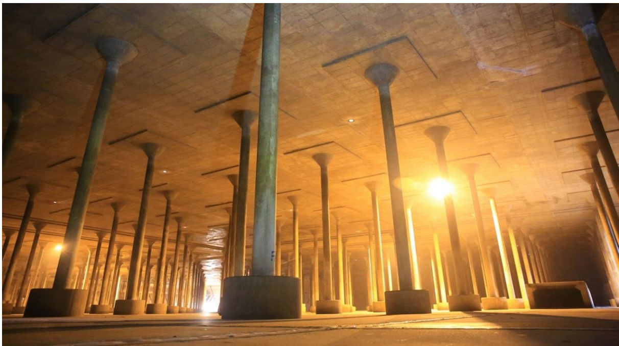
Figure 3.2: Typical interior of a Rand water reservoir
