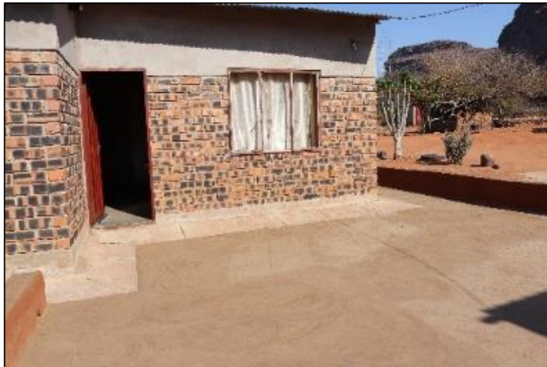
Figure 18: A standard RDP house provided by the government.
