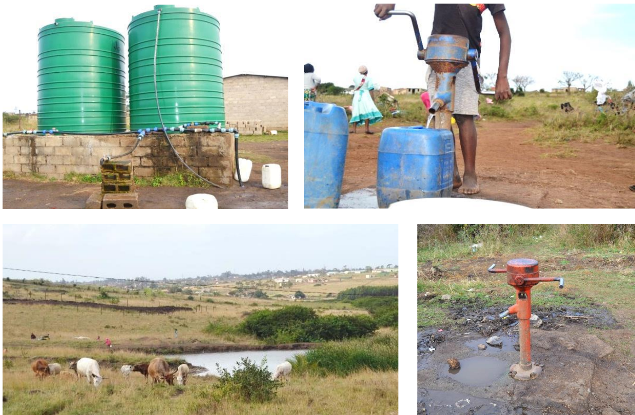
Figure 4.9 (top left): JoJo water tanks where there is a borehole, which pumps the water to the tanks in Nkombose, (top right): A boy from the Ogengele community paddling the hand-operated lever pump for water, (bottom left): A small dam in Nkombose where some residents get water, (bottom right): A hand-operated lever pump in Ebaswazini.
