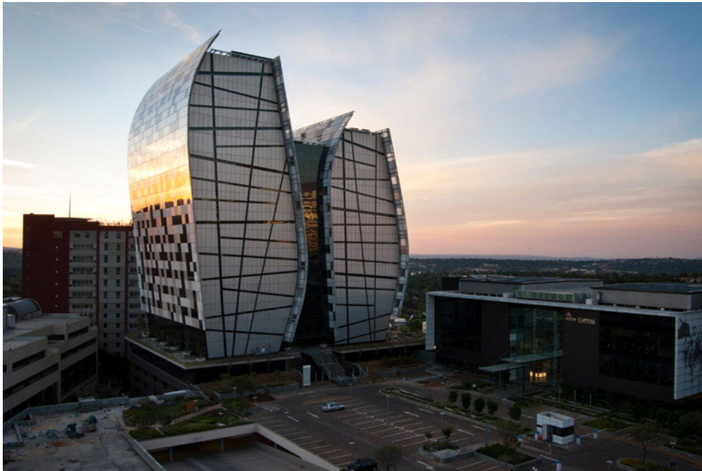
004. Norton Rose Fullbright (2010), Sandton, Paragon Architects - one of the top Law Firms students apply to.
