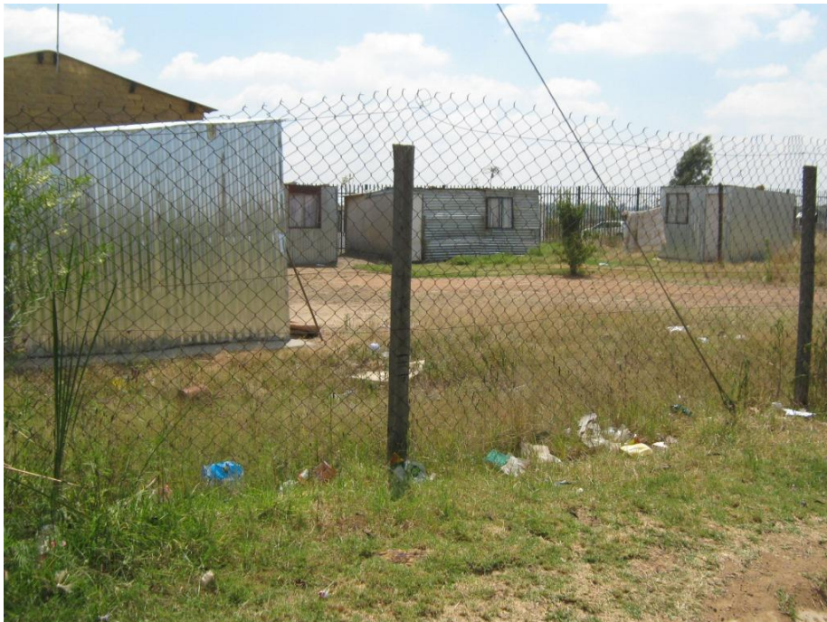
Figure 9: A corrugated iron sheet house in an informal housing area
