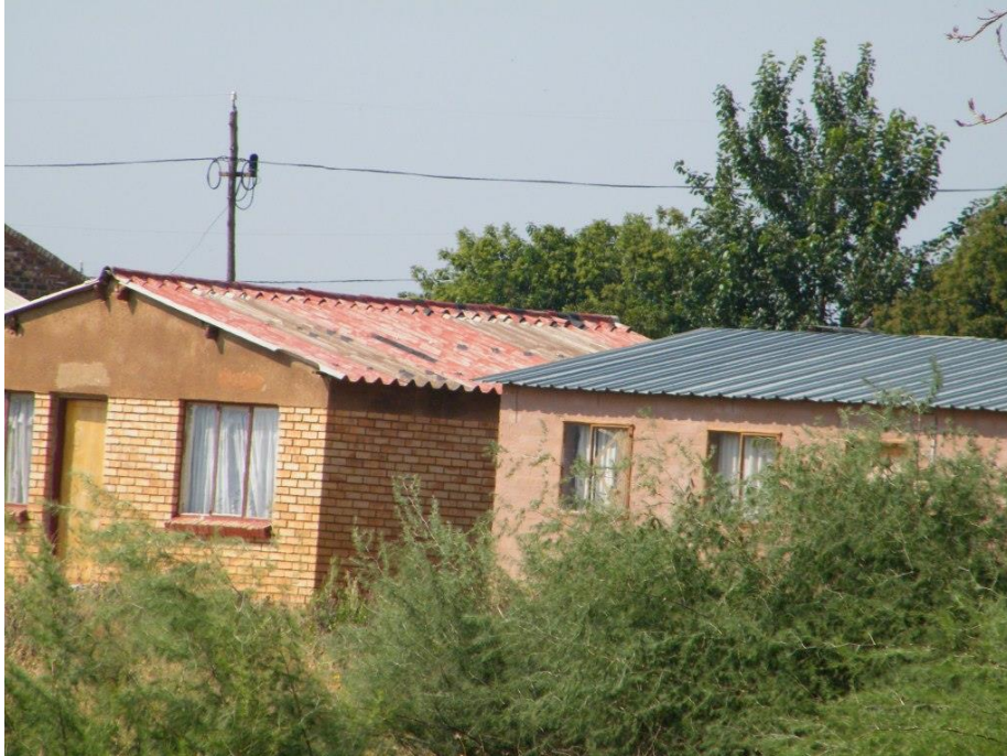
Figure 8: A brick house in a formal housing area
