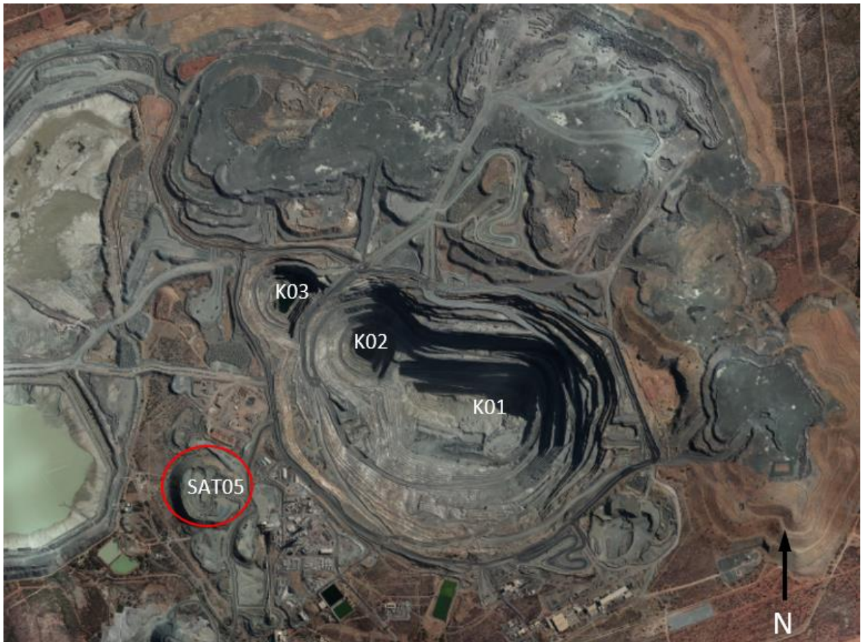
Figure 2-2: Site map of Venetia Mine showing location of satellite stockpile (Venetia Mine, 2019).
