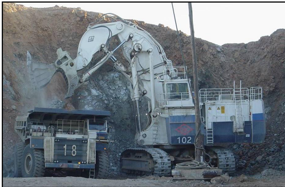
Figure 5.14 RH200 face shovel loading a blasted muckpile into a haul truck
