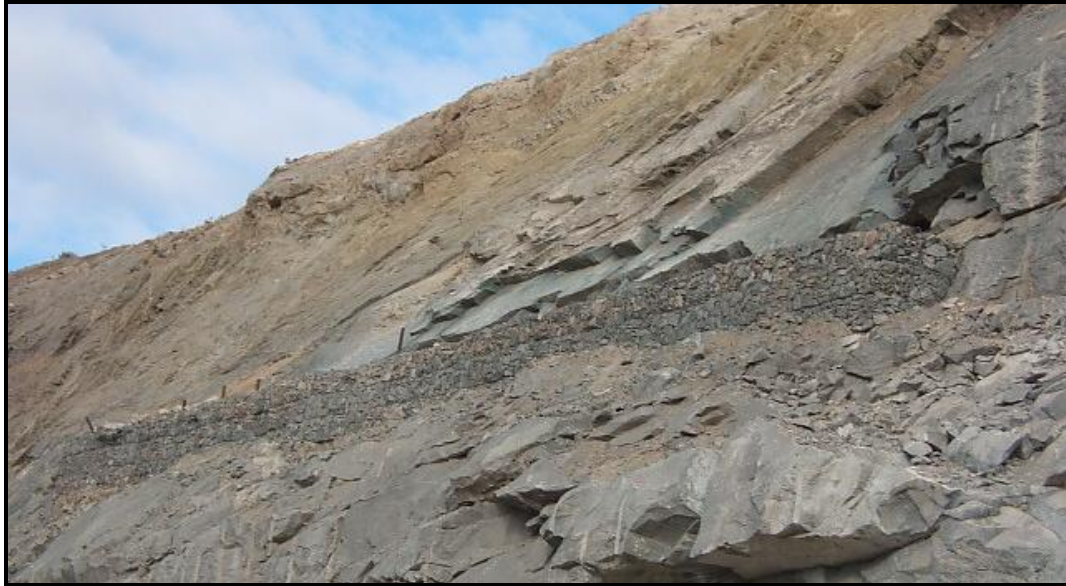
Figure 8.17 Gabion wall built below the Bench 11 failure in Sandsloot pit
