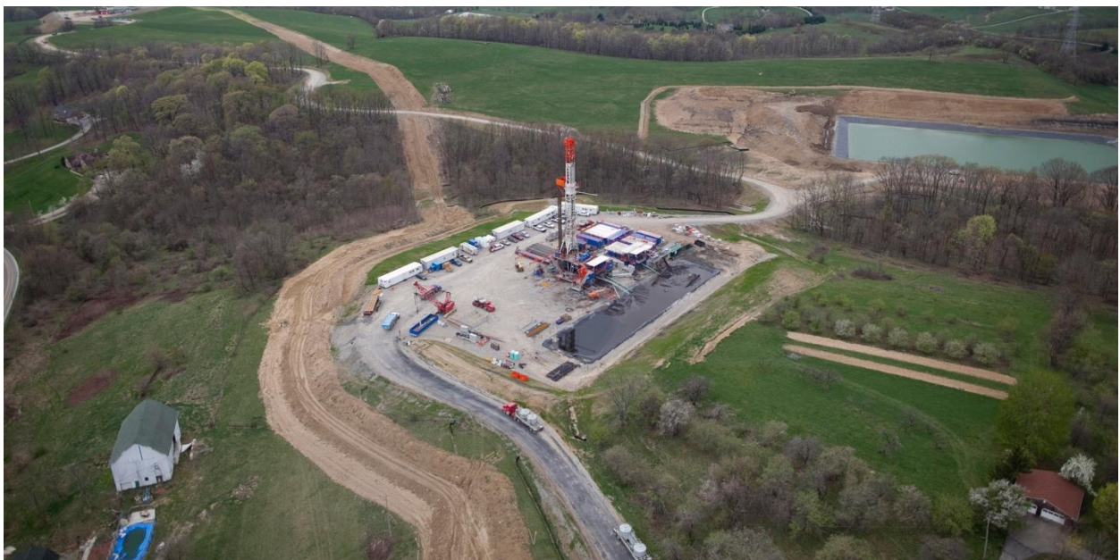
Figure 6.4: A shale gas well site in Pennsylvania, US.
