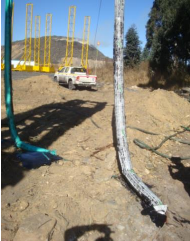
Figure 32: Photo of suspended liners filled with explosives (Taken by Marton, 2011)
