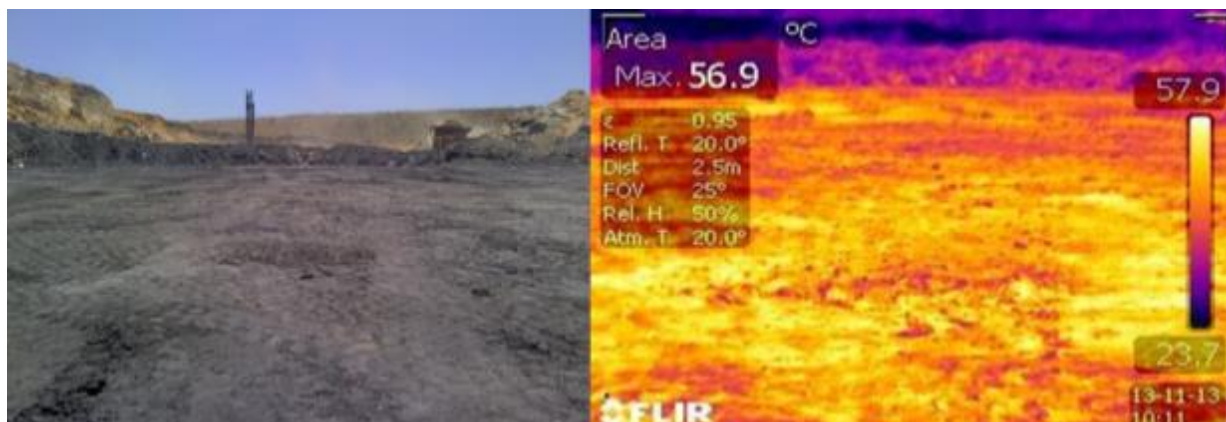
Figure 35: Thermal image of identified risk area at Goedgevonden, 13 November 2013 (photograph taken by Botha, 2013)
