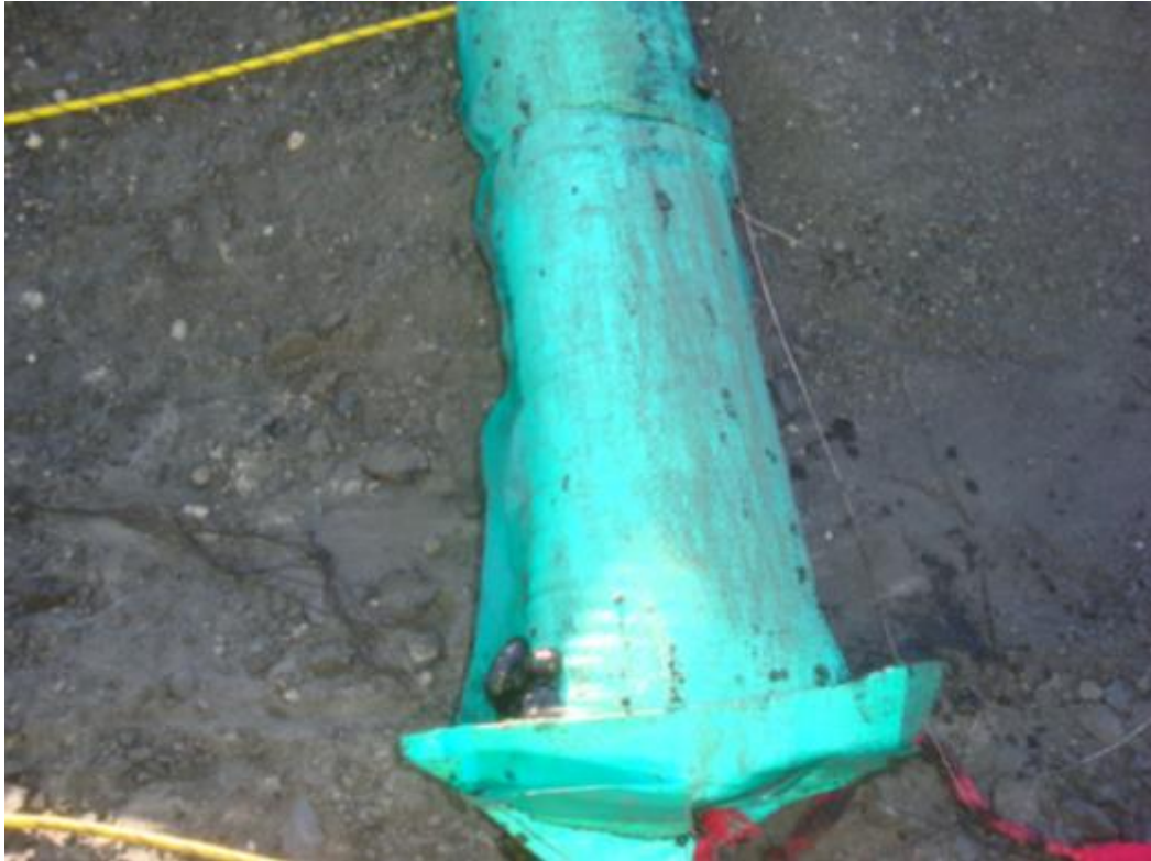
Figure 31: Photo of Liner pulled from pre-split hole (Taken by Marton, 2011)
