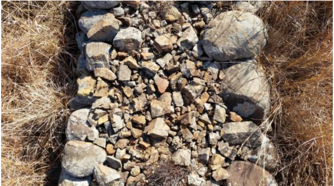
Figure 6.1: Photograph of numerous potshards mixed with stone as infill for wall construction (photograph: Tiffany Henshall)
