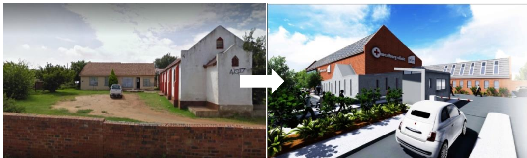
Westbury Clinic before the upgrade Source: Google maps
