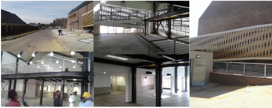
Westbury health care facility upgrade in progress Source: Author, 2016
