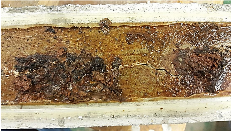
Figure 3.7: Photograph showing crack on surface of concrete
