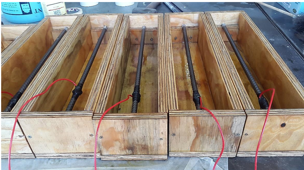
Figure 3.5: Photograph of reinforcing bar (with conductive electrical wire attached) in the formwork mould.
