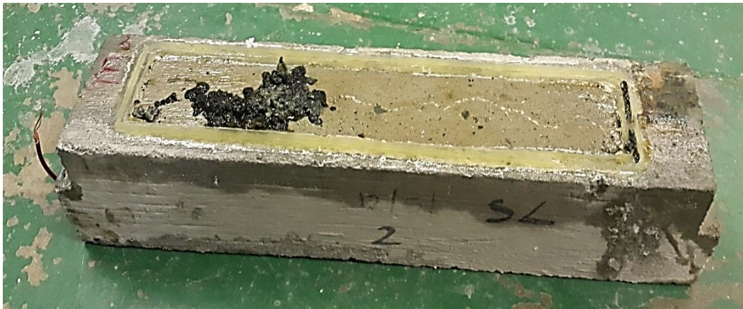
Figure C.3.1: SL #2 prism with corrosion products
