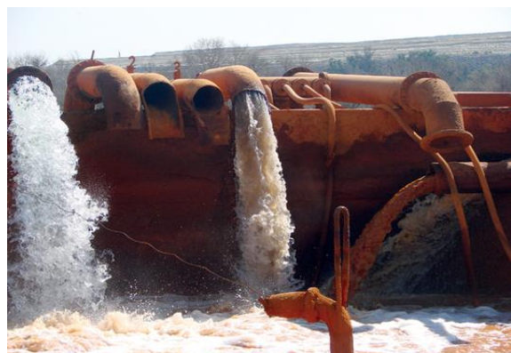
Figure 4A: Water pumps at the Grootvlei Mine in the Eastern Basin prior to the cessation of pumping (du Toit, 2011)
