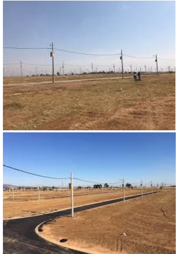
Figure 1.5 Palm Ridge extension 10, Ekurhuleni serviced land. The municipality provides service parcels of land with basic infrastructure for households to build their own housing units with their own resources.
