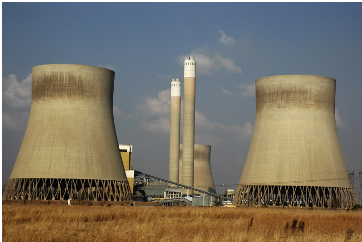
Figure 5: Typical Eskom power station (Image: Graeme Williams. Brand South Africa)
