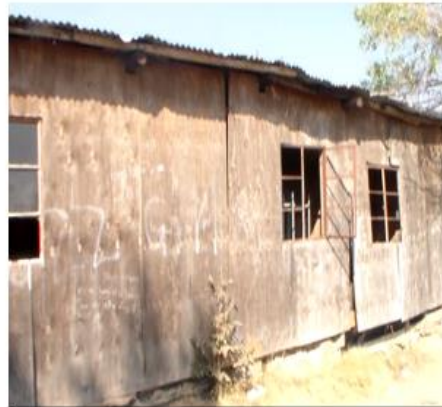
Image 4. An old building structure
