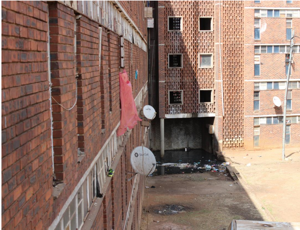
Figure 3. Madala Hostel in Alexandria (Source-Authors own photograph taken on 25 th April 2017)
