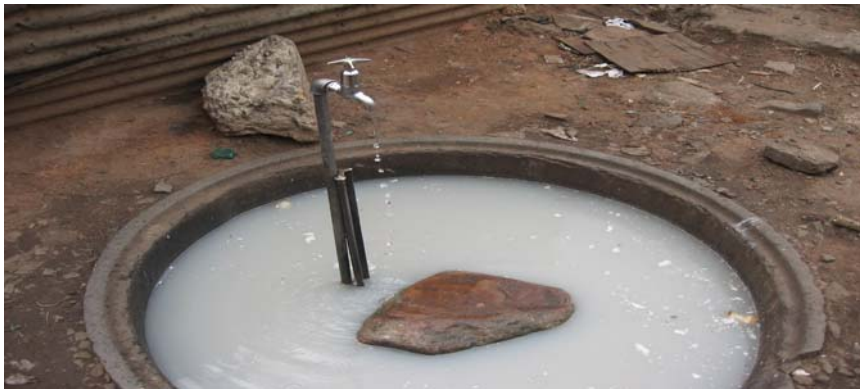
Figure: 7 Water tap with contaminated water
