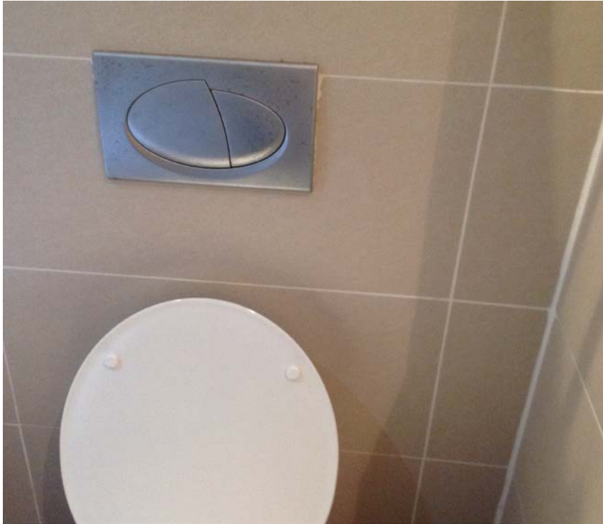
Figure 21: Low Water Toilet Flushing System
