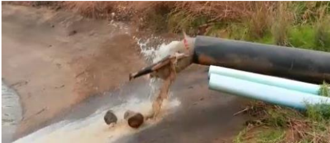
Figure 5-2: Exit of the 435 mm Ø Medium Duty Foam Pig and the Removal of Debris
