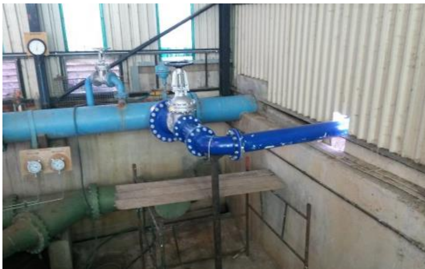
Figure 4-9: Installation of New 200 mm Launching Kicker Line
