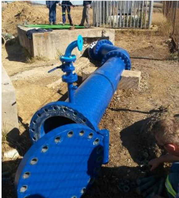
Figure 4-8: Installation of New Pig Launcher
