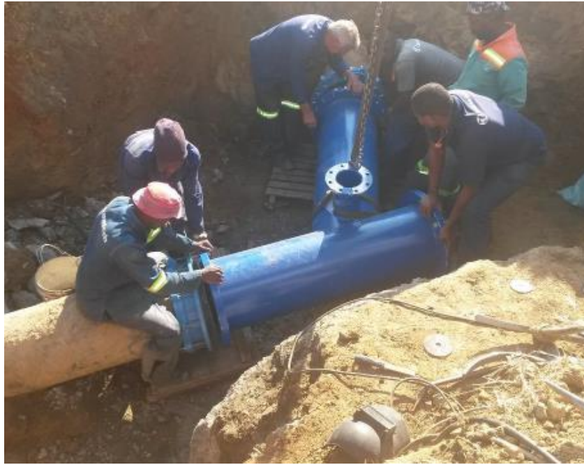
Figure 4-10: Installation of New Branched Tee Piece
