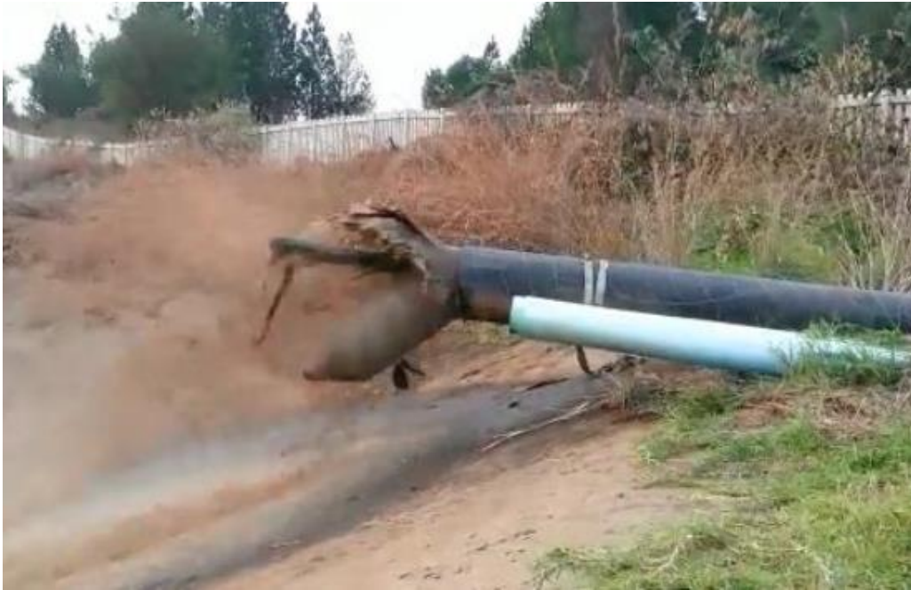
Figure 5-4: Exit of the 440 mm Ø Medium Duty Foam Pig and the Removal of Debris
