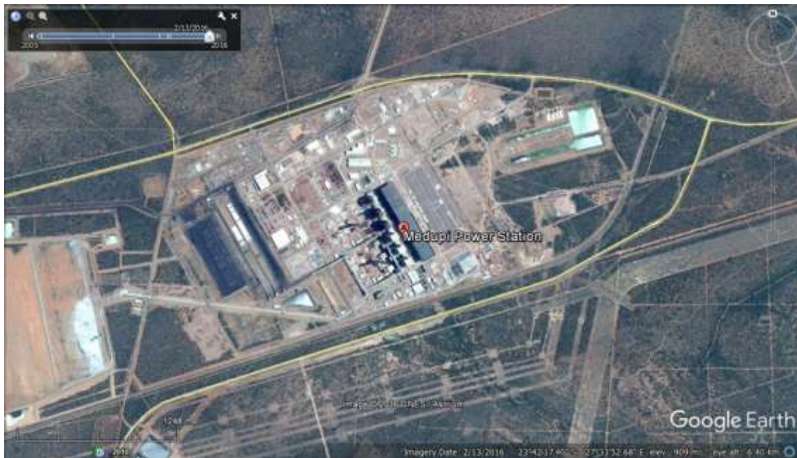
Figure A2: Aerial photographs of Medupi PS in 2005 and in 2016 ( https://www.google.com/earth )
